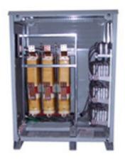
It is a purely passive equipment consisting of a single inductor combined with a relatively small bank of capacitors
